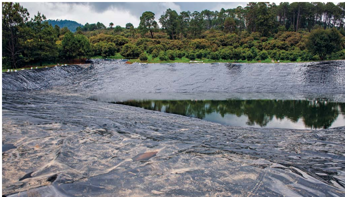
Plastic tubs to store water that industrial avocado cultivation needs in enormous quantities.
